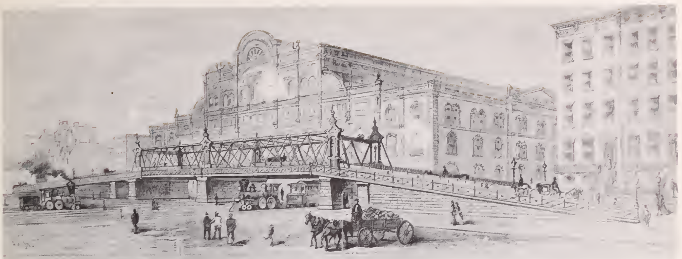
Fig. 8. North facade of the train shed, Grand Central Depot, c. 1888. This view shows a combination pedestrian and vehicular bridge across grade-level tracks.
